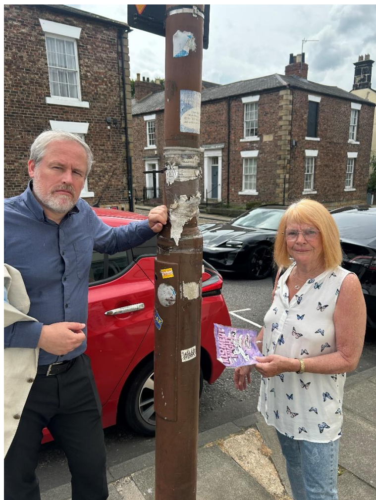
Image 1 – poor condition of lampposts around Durham
